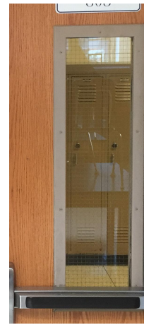
Door with Raised Steel Molding
